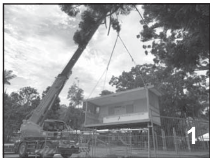
The photo sequence shows the canteen being lifted, placed on the truck then driven off site.
