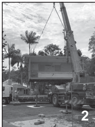
The photo sequence shows the canteen being lifted, placed on the truck then driven off site.
